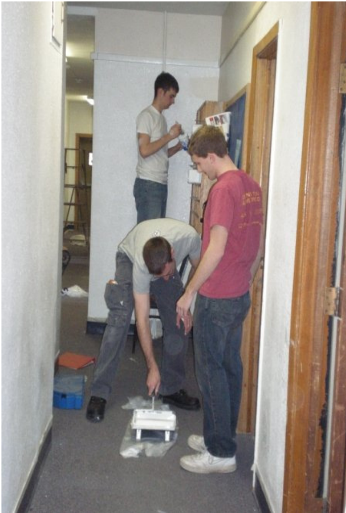
Kyle Cokeley, Dan Falk, Nick Goedkin painting the first floor hallway.
